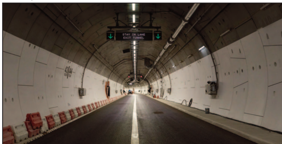
Tunnel Interior - Credit - Riverlinx/TfL
