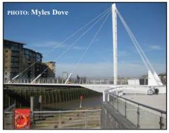
It can open up for river traffic to enter or leave Deptford Creek, when the bridge is turned to point northwards towards the Isle of Dogs, pivoting where a tall post at one end has suspension cables fixed to it.
